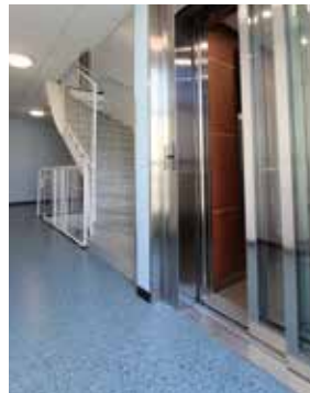
Elevator installed next to stairwell.
