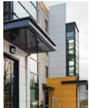
Elevator installed inside stairwell, stairs moved outside.
