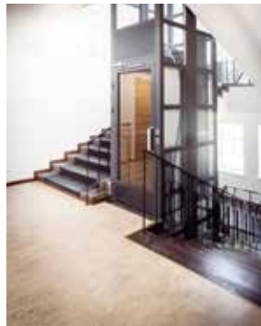
Elevator installed inside the stairwell.
