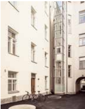
Elevator installed outside the building in an external shaft.
